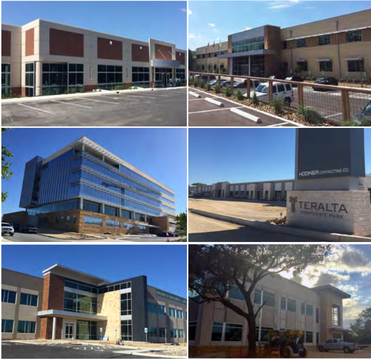
Clockwise from top left: University Oaks IV, GM Financial Campus, Landmark One, Teralta, One51 Phase II, Bella Vista.
